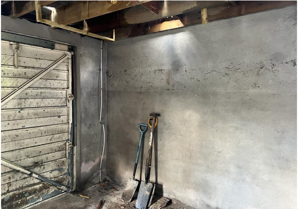
Richill before and after (Garage to Kitchen)
