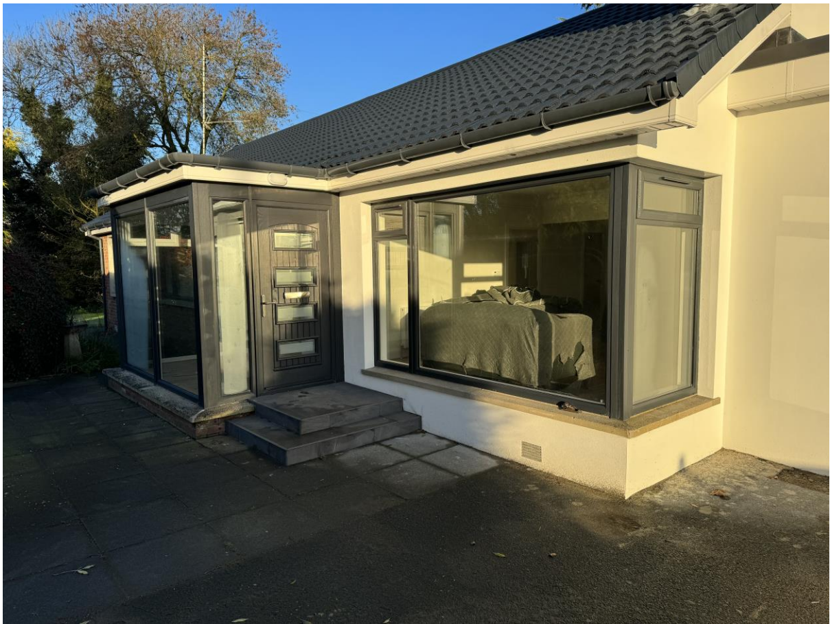
Richill before and after (Front Elevation)
