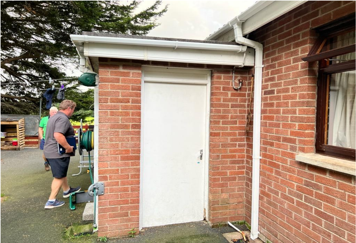
Richill before and after (Garage to Kitchen)
