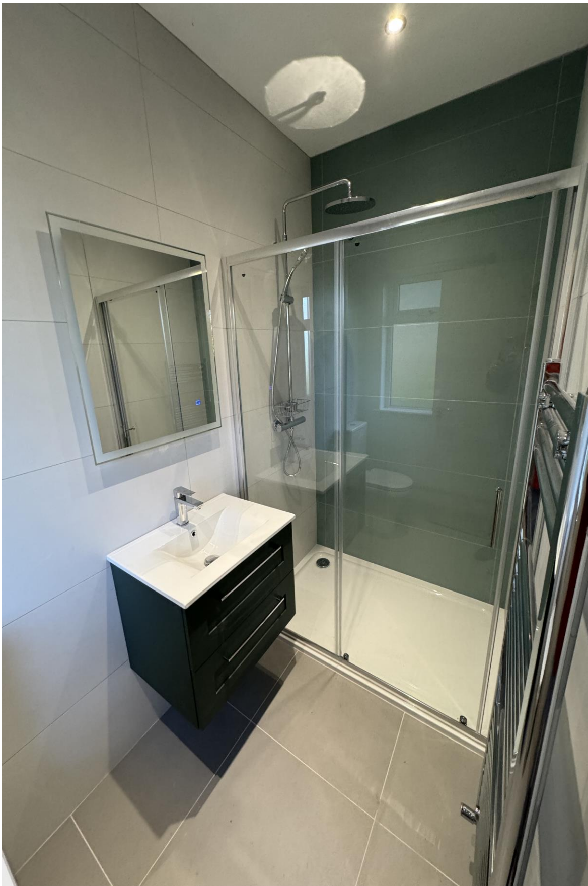
Richill before and after (Ensuite)
