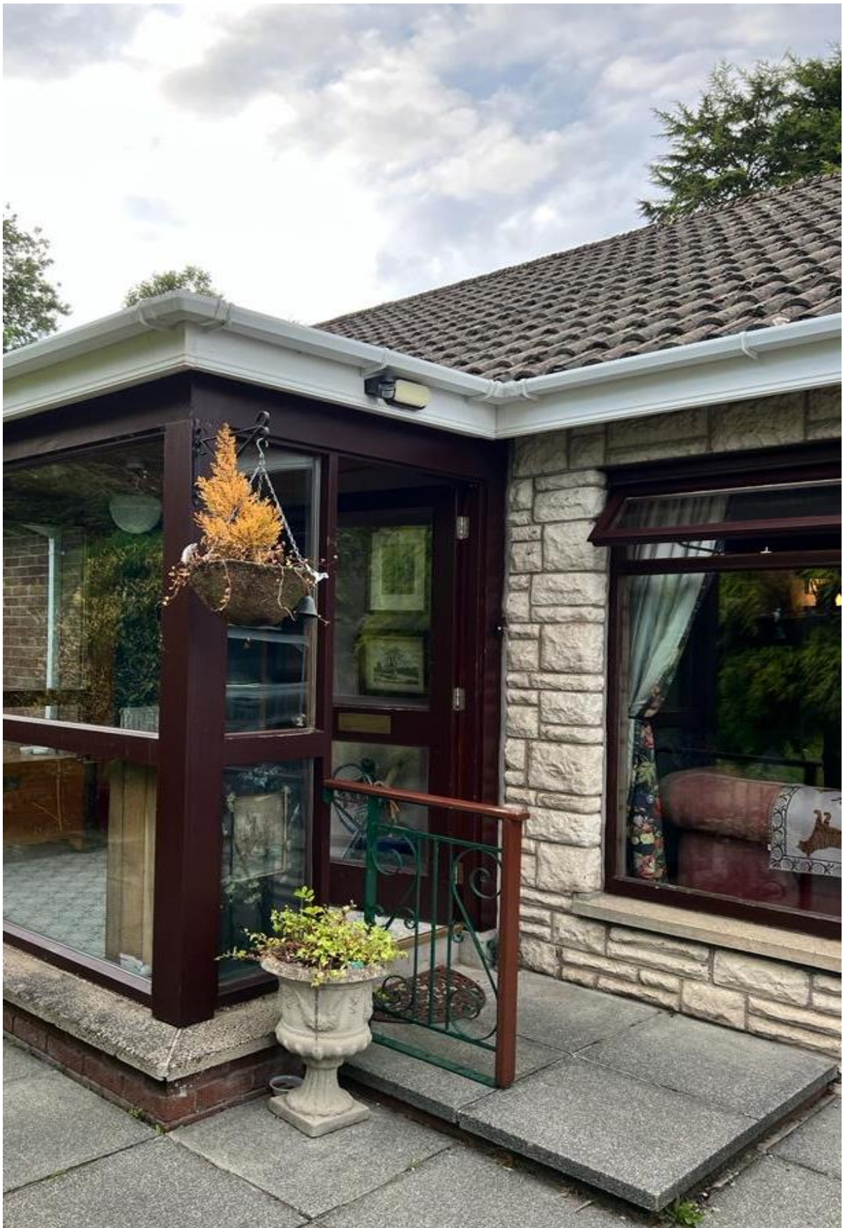
Richill before and after (Front Elevation)
